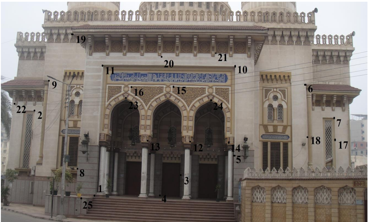
Figure (5) The distribution of observed points on EL-NASR Mosque façade
